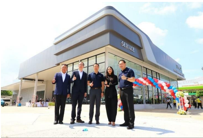
Exhibit 13: BYD showroom by SUSCO Beyond
