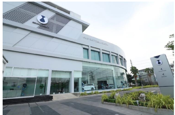
Exhibit 14: DENZA showroom by SUSCO Beyond
